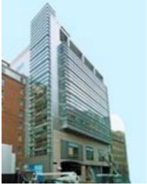
Main South building
