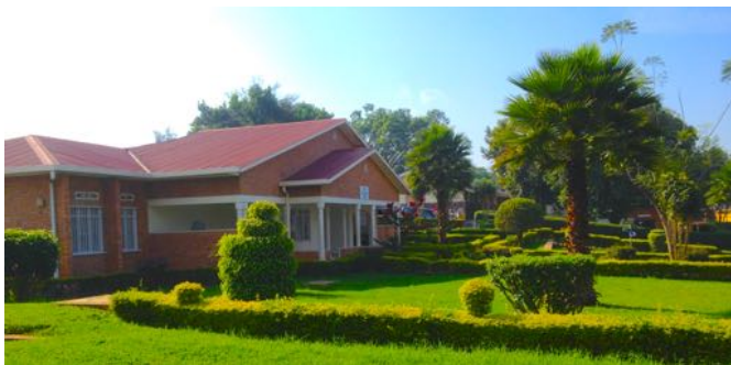
Central Hospital University of Kigali, Rwanda
